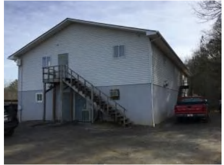
3). Northwest Elevation - Feb 07, 2017
