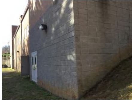
2). East Elevation - Feb 08, 2017
