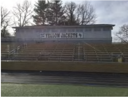
1). East Elevation - Feb 27, 2017
