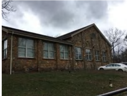
2). North Elevation - Jan 17, 2017
