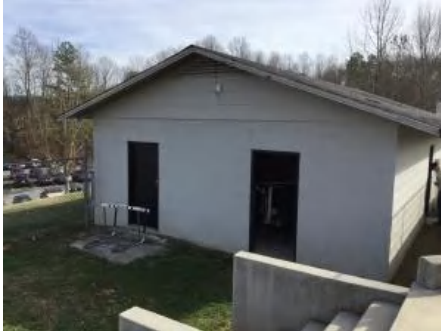
1). North Elevation - Feb 08, 2017
