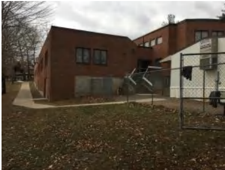
4). Northwest Elevation - Jan 23, 2017
