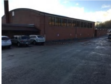
2). Northwest Elevation - Feb 09, 2017
