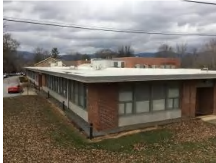
2). Southwest Elevation - Feb 09, 2017
