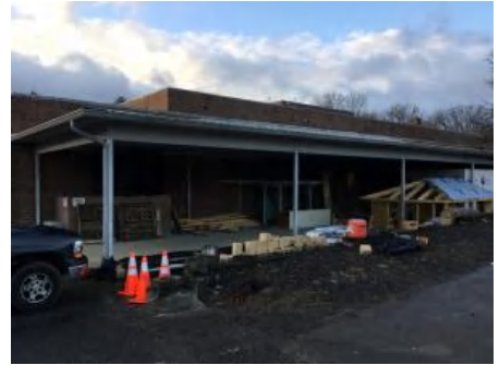
3). North Elevation - Jan 27, 2017
