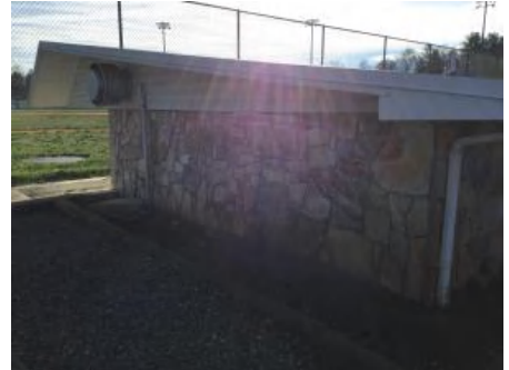
3). North Elevation - Jan 24, 2017
