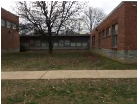
4). East Elevation - Feb 09, 2017
