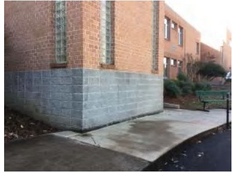
3). North Elevation - Feb 08, 2017
