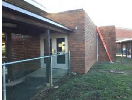
2). West Elevation - Feb 23, 2017
