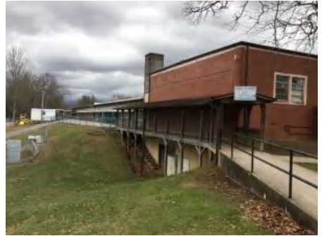
3). North Elevation - Jan 23, 2017
