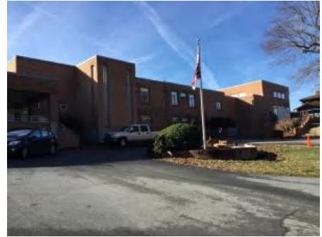
3). North Elevation - Jan 24, 2017
