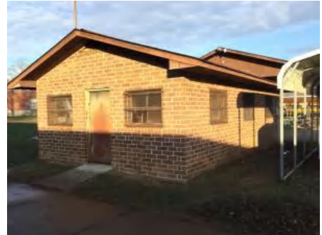
3). Southwest Elevation - Jan 30, 2017
