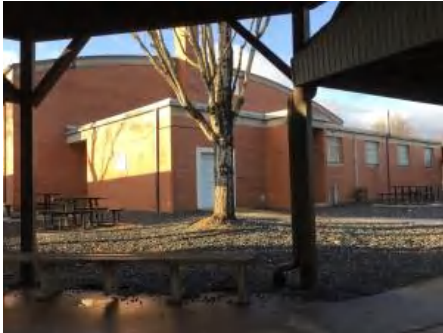
1). North Elevation - Feb 09, 2017
