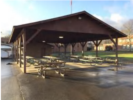
1). North Elevation - Jan 30, 2017
