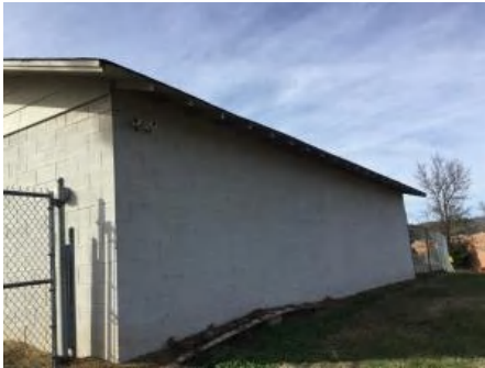
4). South Elevation - Feb 23, 2017
