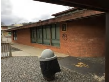
1). North Elevation - Jan 17, 2017
