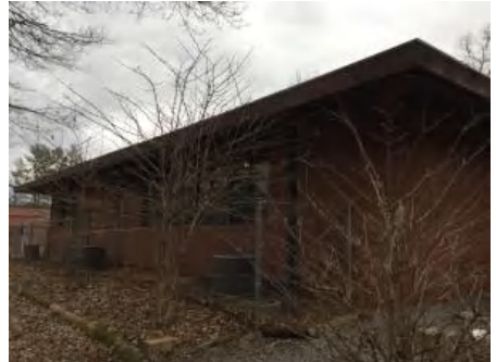
3). North Elevation - Jan 23, 2017
