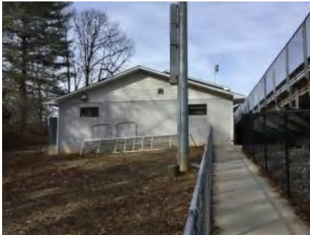
4). South Elevation - Feb 07, 2017
