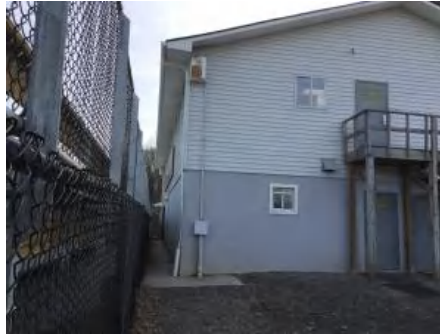
2). Northeast Elevation - Feb 07, 2017
