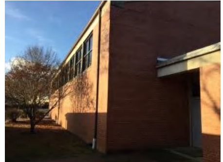
3). East Elevation - Feb 09, 2017
