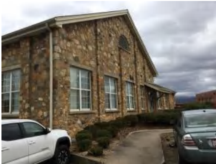
4). South Elevation - Feb 15, 2017
