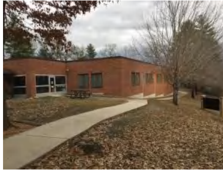
2). Southwest Elevation - Jan 23, 2017
