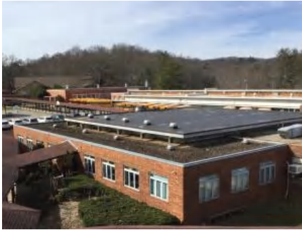
1). South Elevation - Feb 27, 2017
