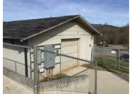
3). South Elevation - Feb 08, 2017
