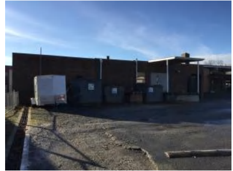
3). North Elevation - Jan 24, 2017
