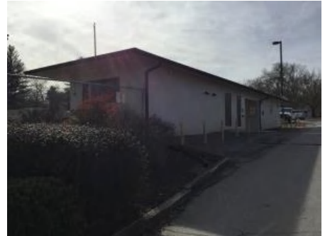
3). North elevation - Jan 30, 2017
