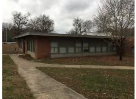
3). South Elevation - Feb 09, 2017
