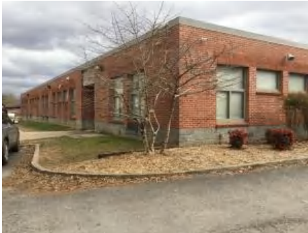
1). North Elevation - Feb 09, 2017
