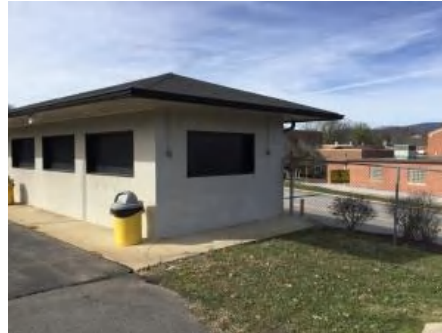
2). West Elevation - Feb 23, 2017
