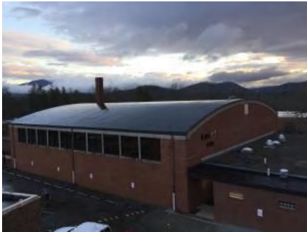
4). Southwest Elevation - Feb 09, 2017
